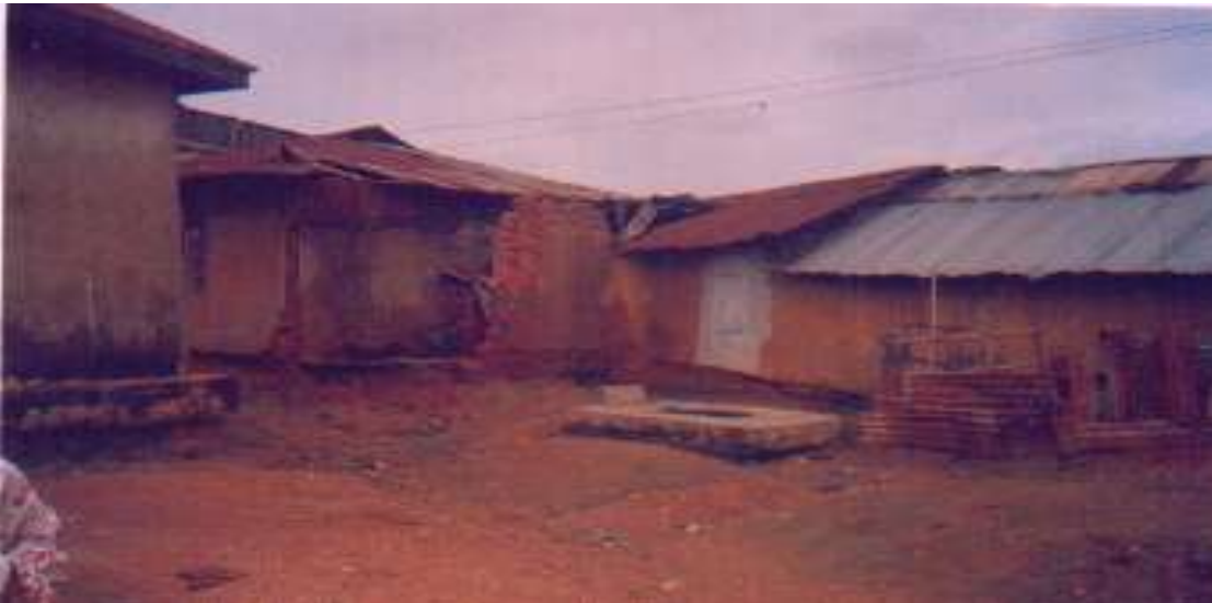
Plate 4:4: Structurally and Qualitatively Deficient Buildings, Jumbled Together in Isale Osun Area
