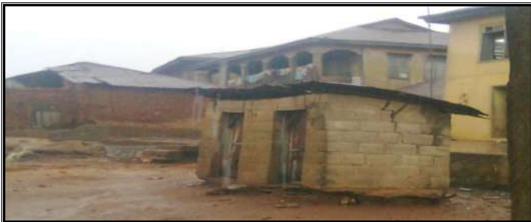
PLATE 4:7: An outdoor Toilet in the Area of Study
