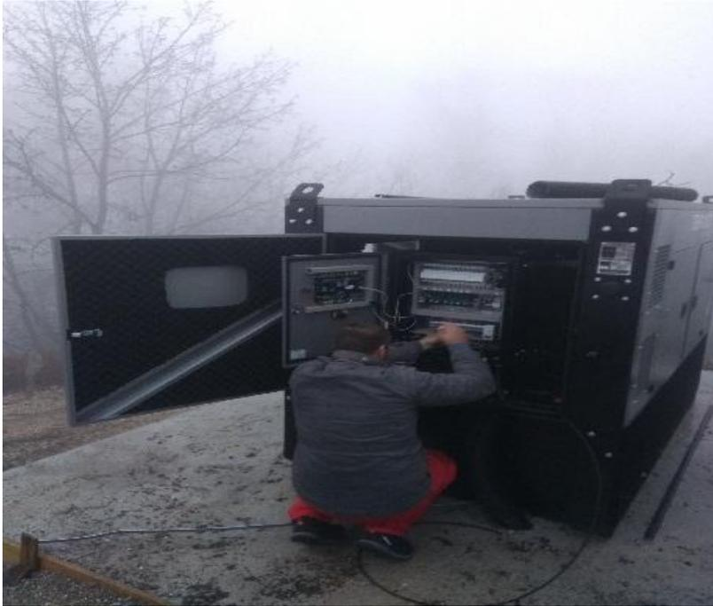
**Figure 2:** Wiring and instalation of diesel generator
